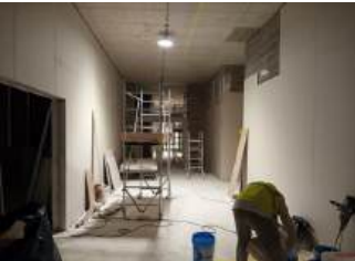
Vista interni / Interior view
