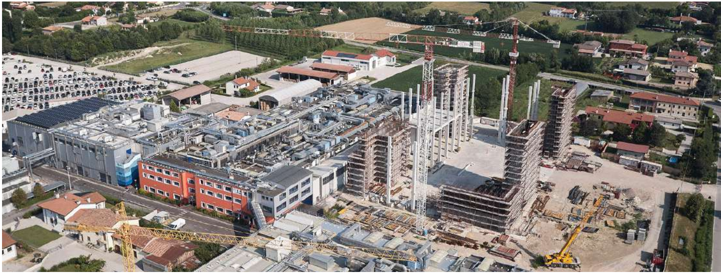
Vista del cantiere del Fabbricato H / View of the construction site of Building H
