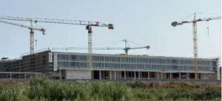
Vista fronte sud / South-facing view
